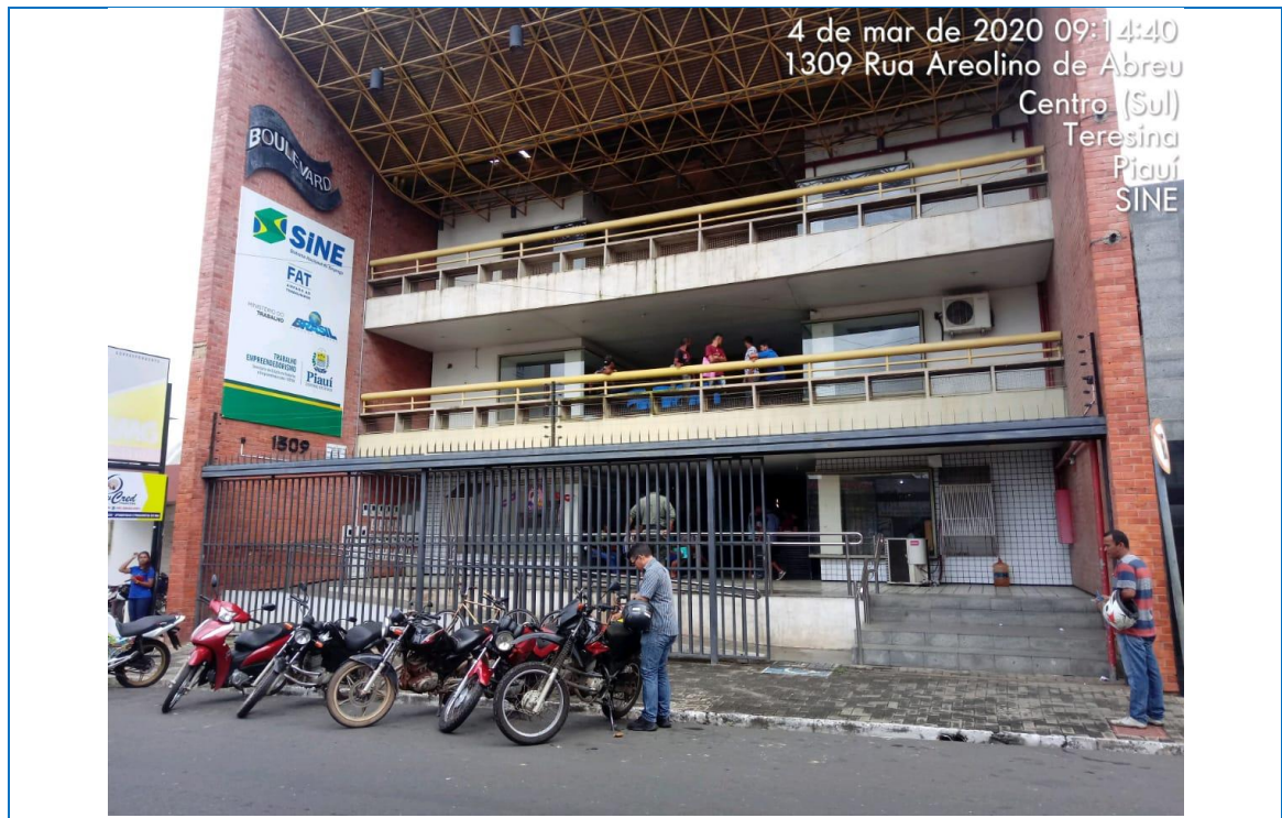
Figura 1 – SINE Boulevard Center - Teresina
