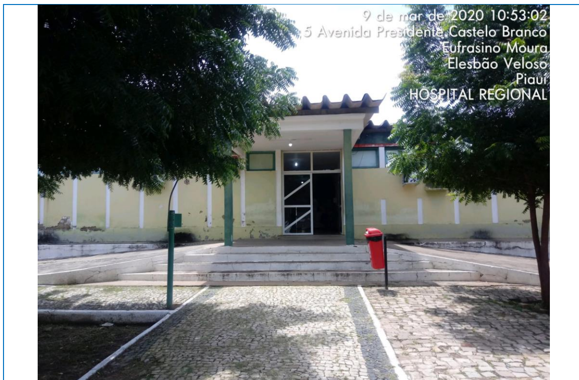
Figura 24 – Hospital Regional – Elesbão Veloso
